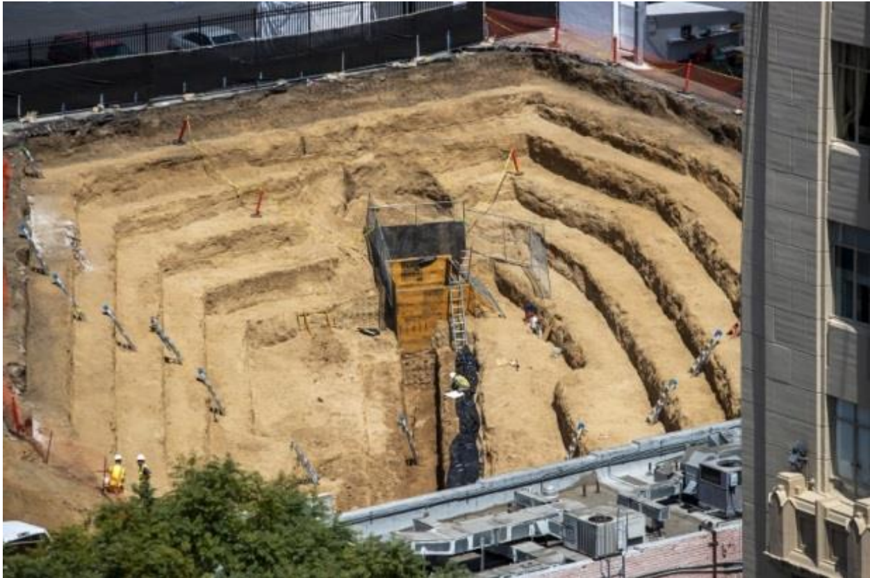
A giant trench is being dug next door to the Capitol Records building to determine if an earthquake fault runs under the site. (Brian van der Brug/Los Angeles Times)
